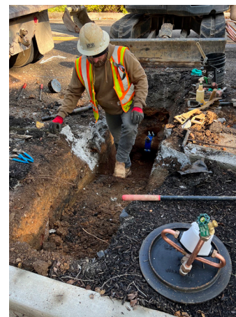
Installing the underground vault for water spigot.
